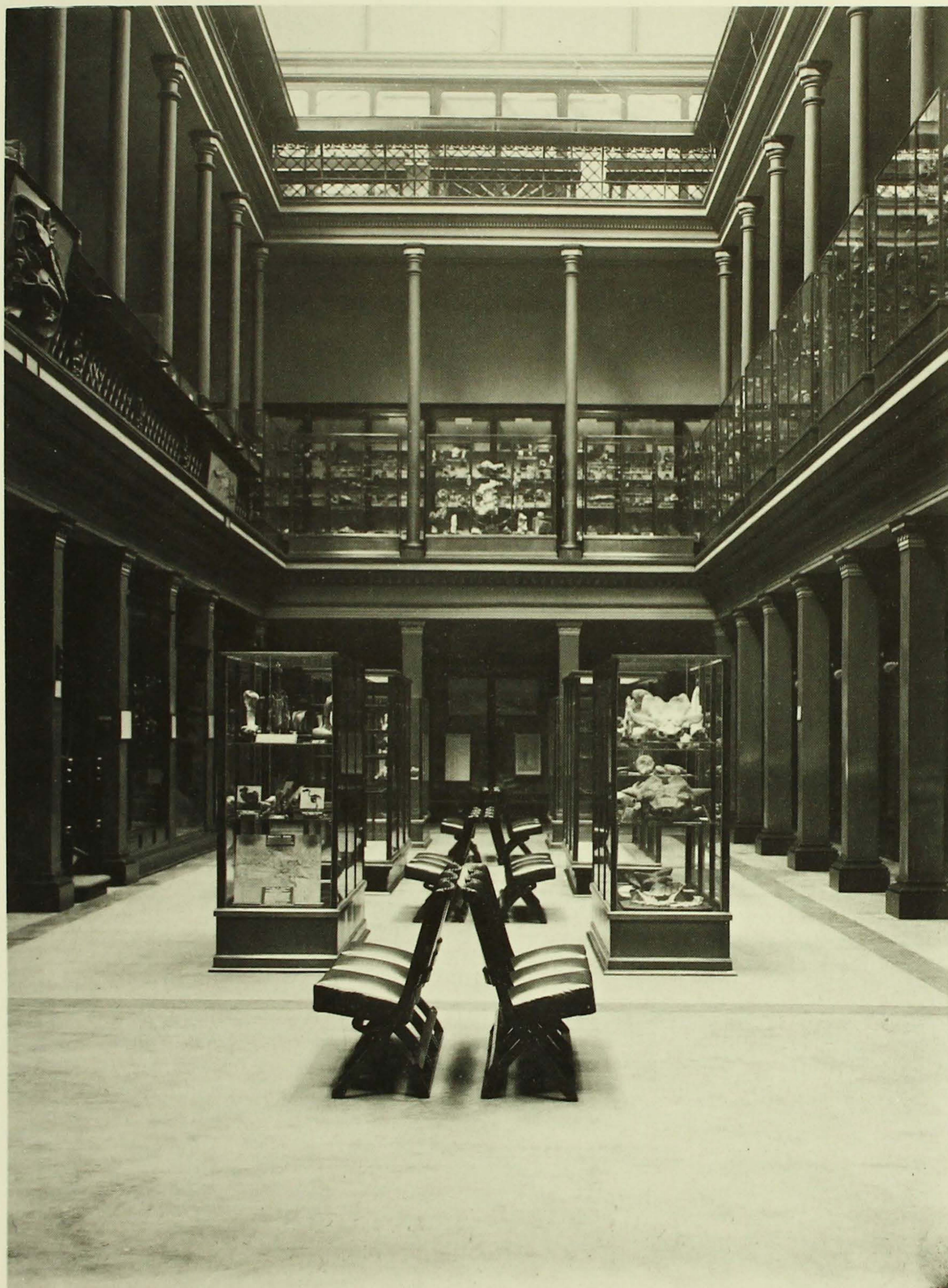
The Long Galley, looking towards the east, early twentieth century, showing the third floor (added in 1890) and a considerable reduction in clutter.
