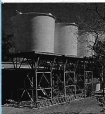
Increased header tank storage at the Sir John Proud Aquarium
