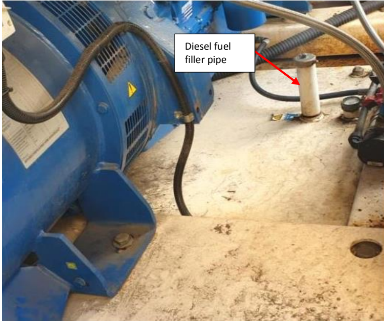
Figure 5 - location of diesel fuel filler pipe
